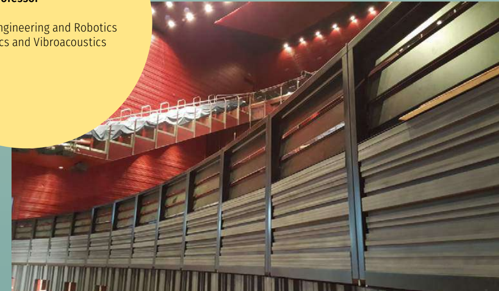
The frontal wall of the orchestra pit in the Krakow Opera – sound screening and reflection by the elements of the barrier
